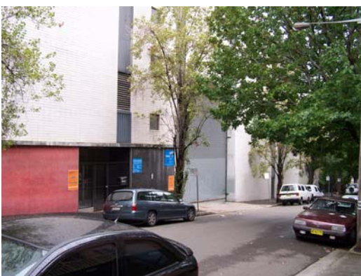
Substation Tx Entrance
